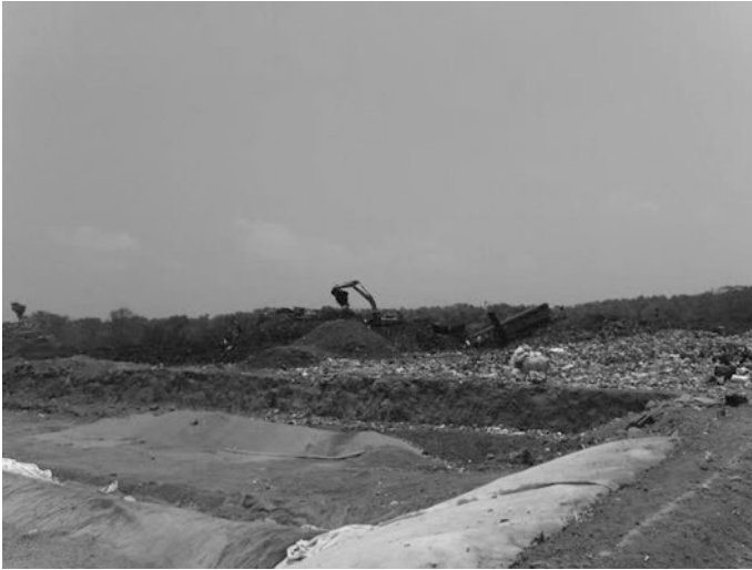
Fig. 1 Landfill construction at Saligao
